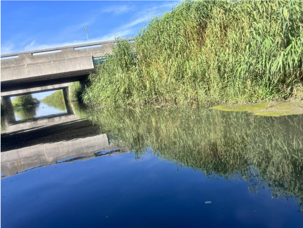
Photograph 10: View beneath the Otto Du Plessis Bridge. The proliferation of reeds along the edges of the channel can be seen; likely the result of loading of nutrient-enriched inflows into the lagoon.
