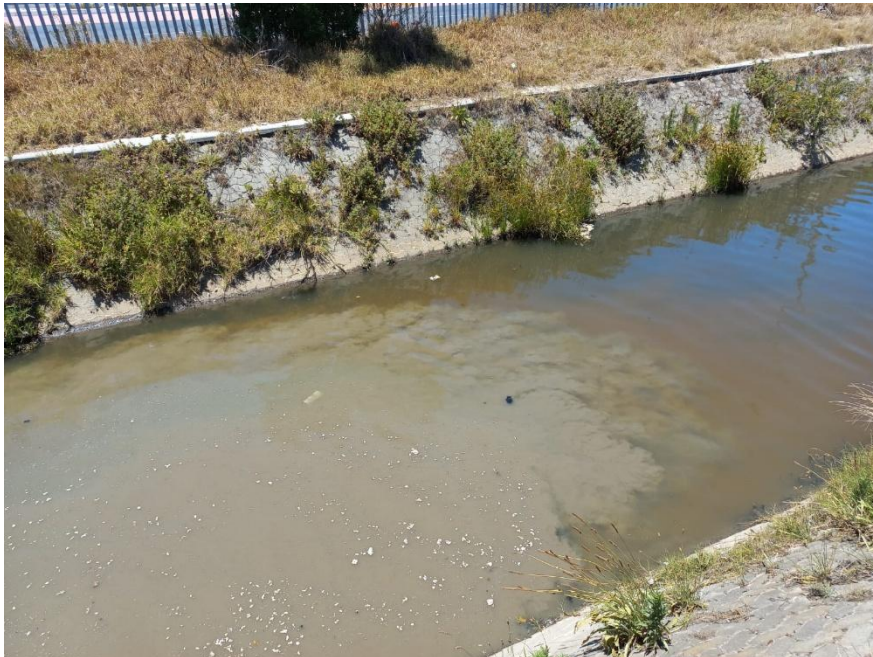
Photograph 24: Pollution loading from the Theo Marais Canal outlet pipe and discharged wastewater (upstream of the site) is pictured in this image.
