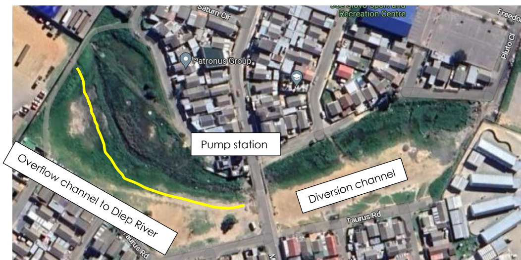
Figure 9-3. Aerial view of the Milky Way channel showing the diversion channel and sewer pump, and overflow downstream of Milky Way Drive. Yellow line indicating potential position to install low flow biofilter channel
