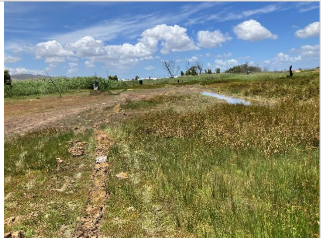
Photo 2-2. Ponding of water on Diep River floodplain – water collects downstream of open drains from the informal settlements
