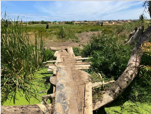
Photo 2-1. Pedestrian crossing over permanent main channel of the Diep River (site Diep 1) upstream of main inflows from Du Noon and associated informal settlements - note dwellings on floodplain in background
