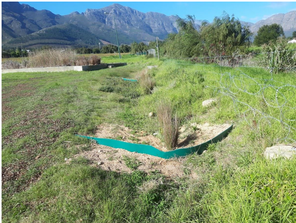
Photo 9-2. A vegetated swale structure post treatment at the Water Hub provides a final polishing phase with low v-notch weirs that are designed to aerate the water before it is discharged into the river alongside (DO 5 -6 mg/l at point of discharge).
