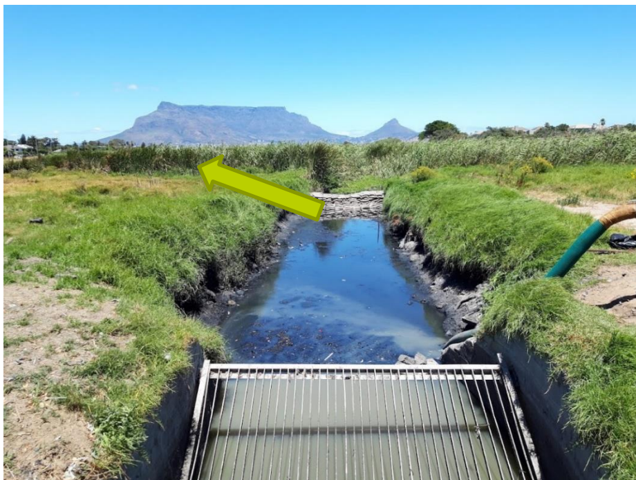
Photo 9-2. Outlet channel near Erica Road which is currently overpumping contaminated water from Joe Slovo and other sources to the sewerage system on the opposite side of Otto du Plessis Drive. Arrow indicates a possible route to an existing low flow channel alongside the road.
