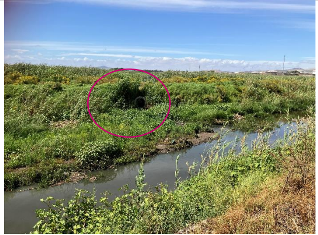
Photo 2-8. Pipe overflow inlet from WWTW reedbeds into Theo Marais channel
