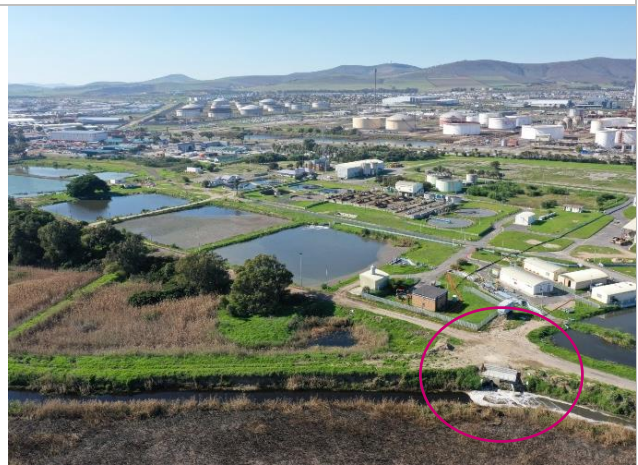
Photo 2-6. Potsdam WWTW showing outlet into bypass channel (circled)
