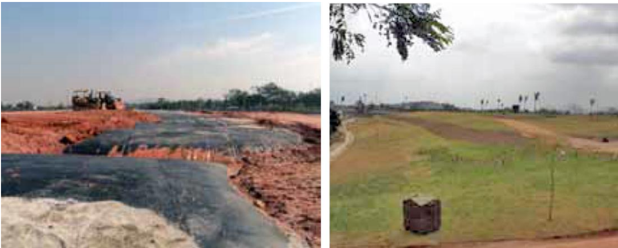
Figure 5-21: An example of Geotextile tubes being covered with topsoil (left) and after vegetation has been established (right).
