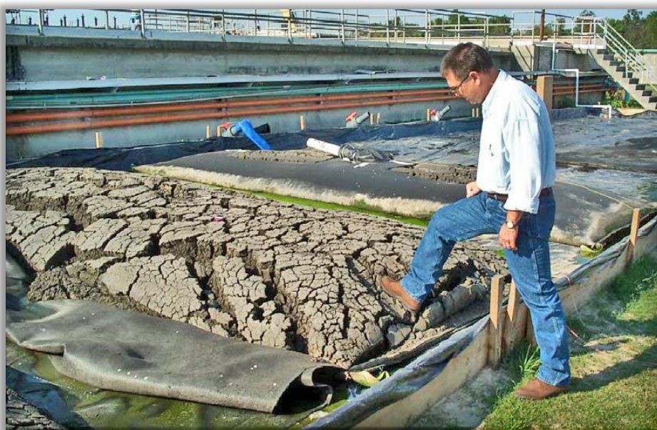
Figure 5-22: Excerpt from Fowler et al (2002): An example of sewage sludge dewatered with the Geotextile tube method indicating material consistency – suitable to be transported by truck.
