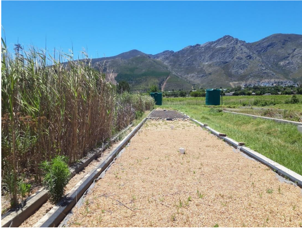
Photo 9-1. Biofiltration cells at the Water Hub. Each cell can be controlled separately or managed as a treatment train. The supply is abstracted from the river and pumped into two 10Kl tanks that feed the cells.
