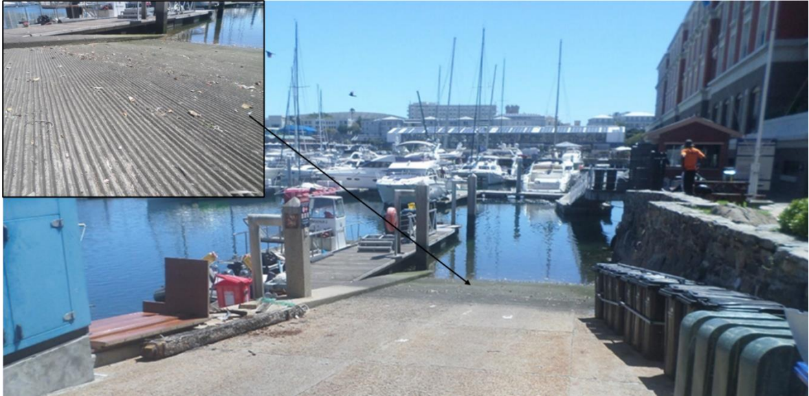
Figure 8-3: Existing V&A Marina Basin slipway.
