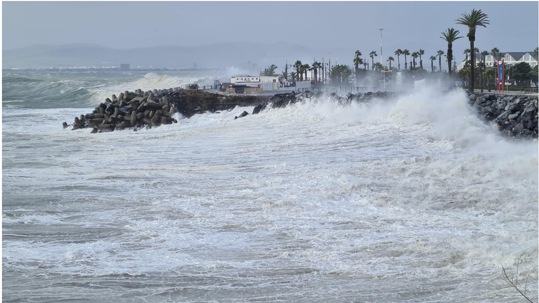
Figure 2-17: Overtopping of rock revetment at approximately 15:00 on 13 July 2020. Photo credit: Stephen Luger.
