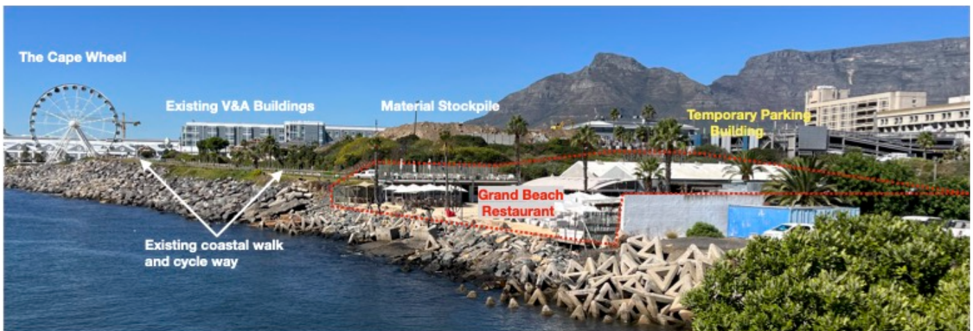
Figure 24 Grand Beach Restaurant in centre of photo with tented structures, umbrellas and beach sand and excavated material stockpile and temporary garage immediately behind (note untidy random coastal protection measures along waters edge.)
