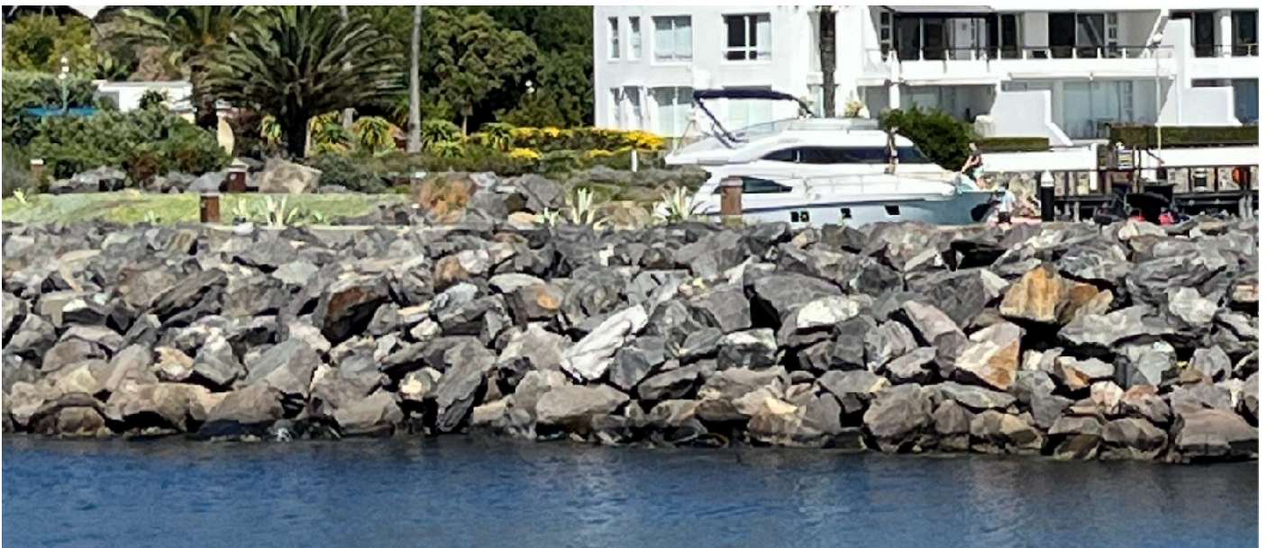
Figure 40 Preferred revetment using large rocks rather than dolos
