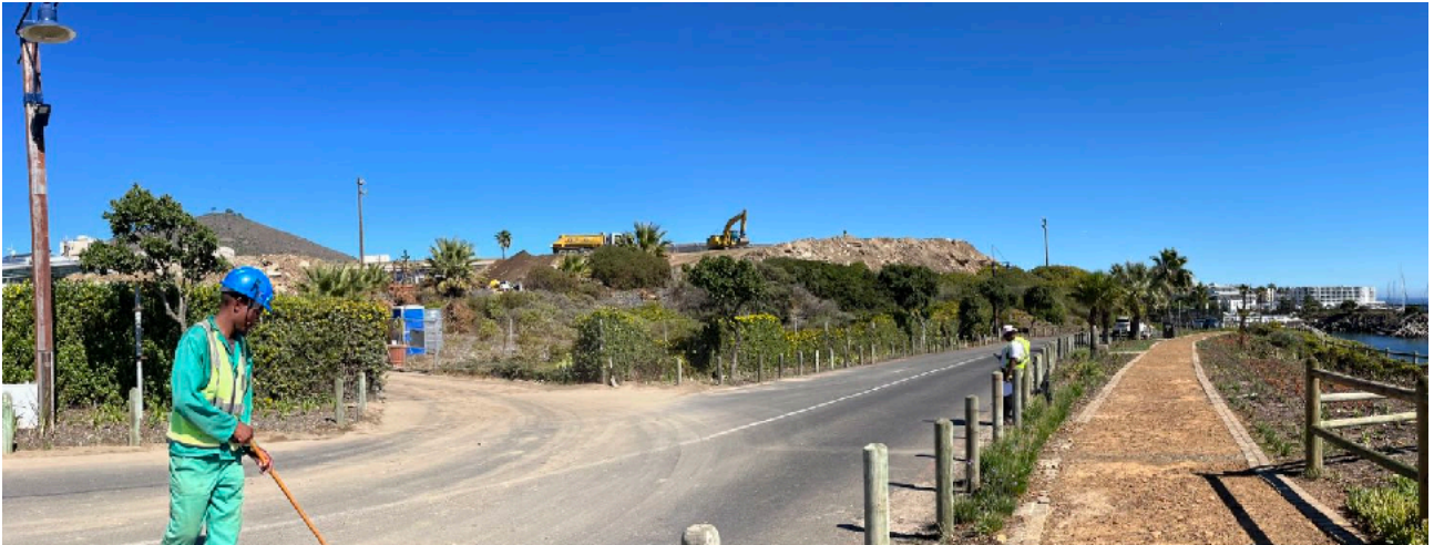
Figure 25 Haul Road between Breakwater Boulevard and Beach Road with pedestrian and cycle path adjacent to the coastal embankment and with landscaped verges including street lighting, timber bollards and fencing and tree, shrub and groundcover planting (note excavated material stockpile to left of road)
